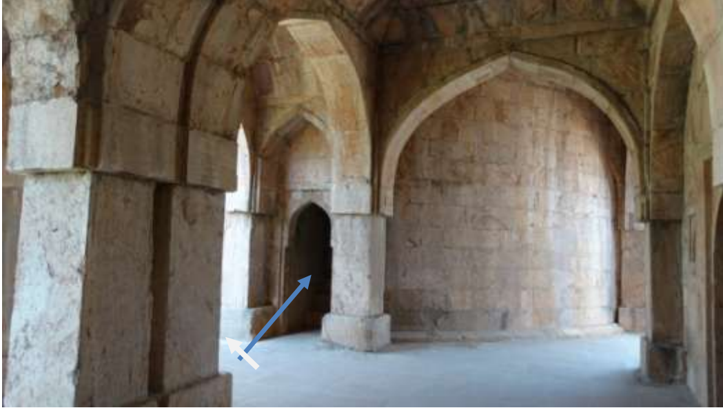
Plate 126 – northern wall of the tower with steps leading to top floor
