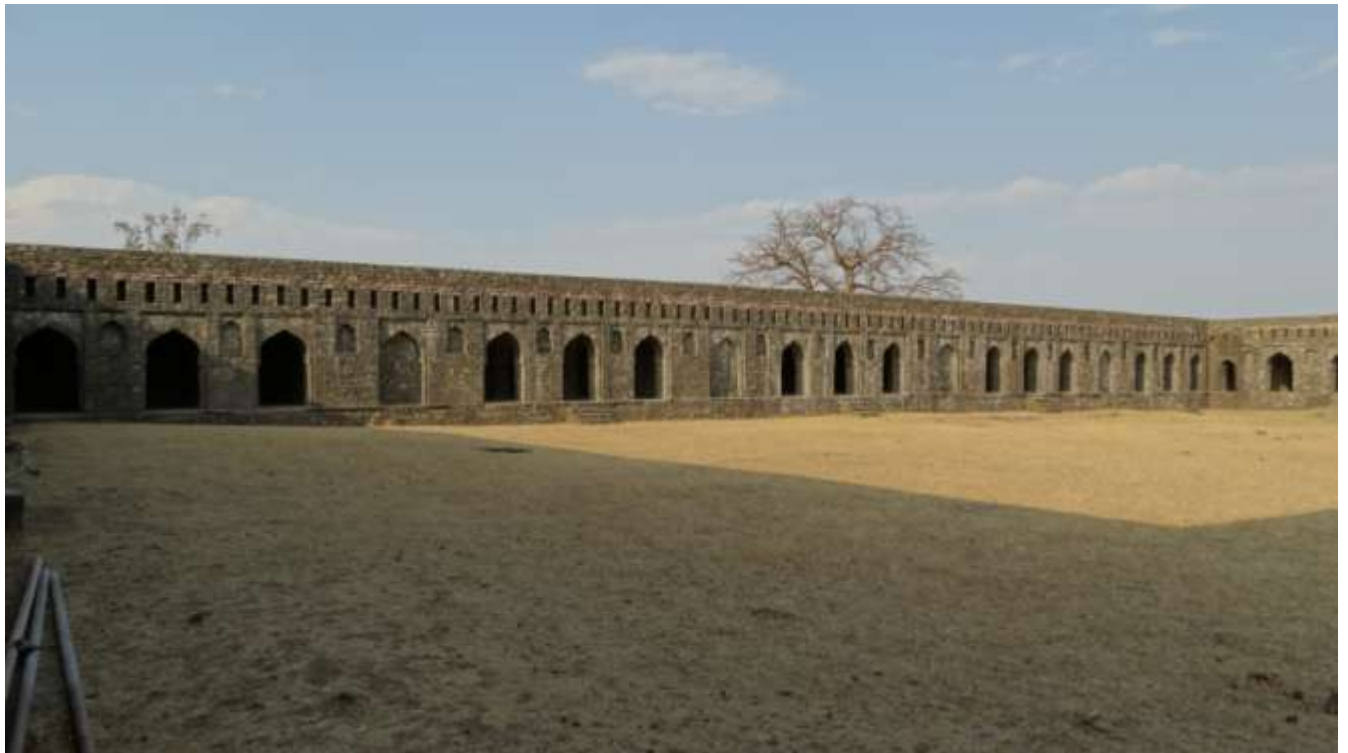
Plate 175 – northern wall of Caravan Sarai
