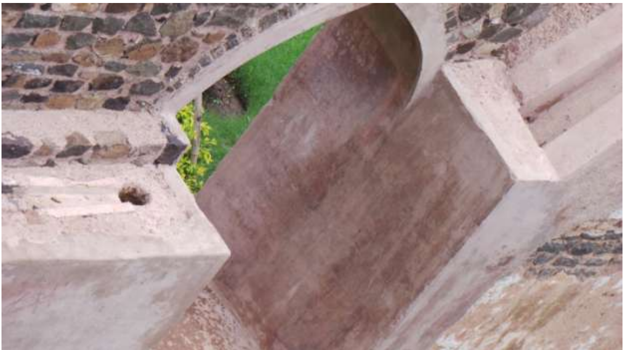
Plate 80 – inbuilt water carrying channels
