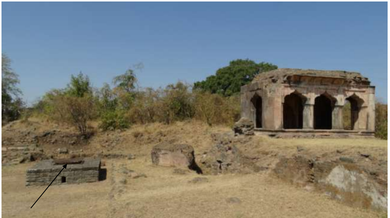
Plate 184 – Sopi Tank and Sopi mosque
