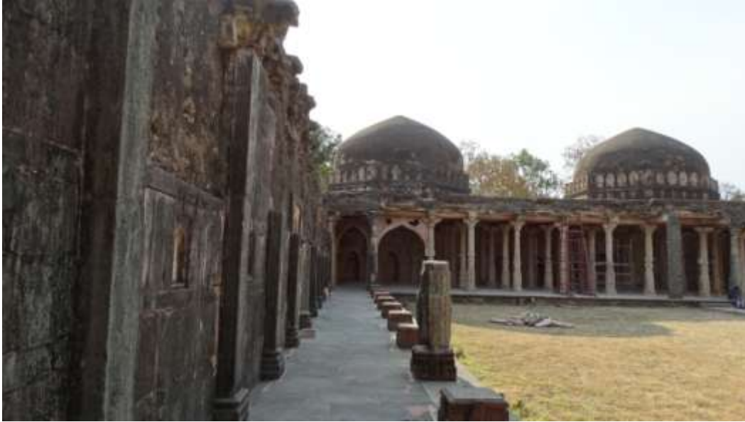
Plate 97 – southern section of inner part of Malik Mughith's mosque
