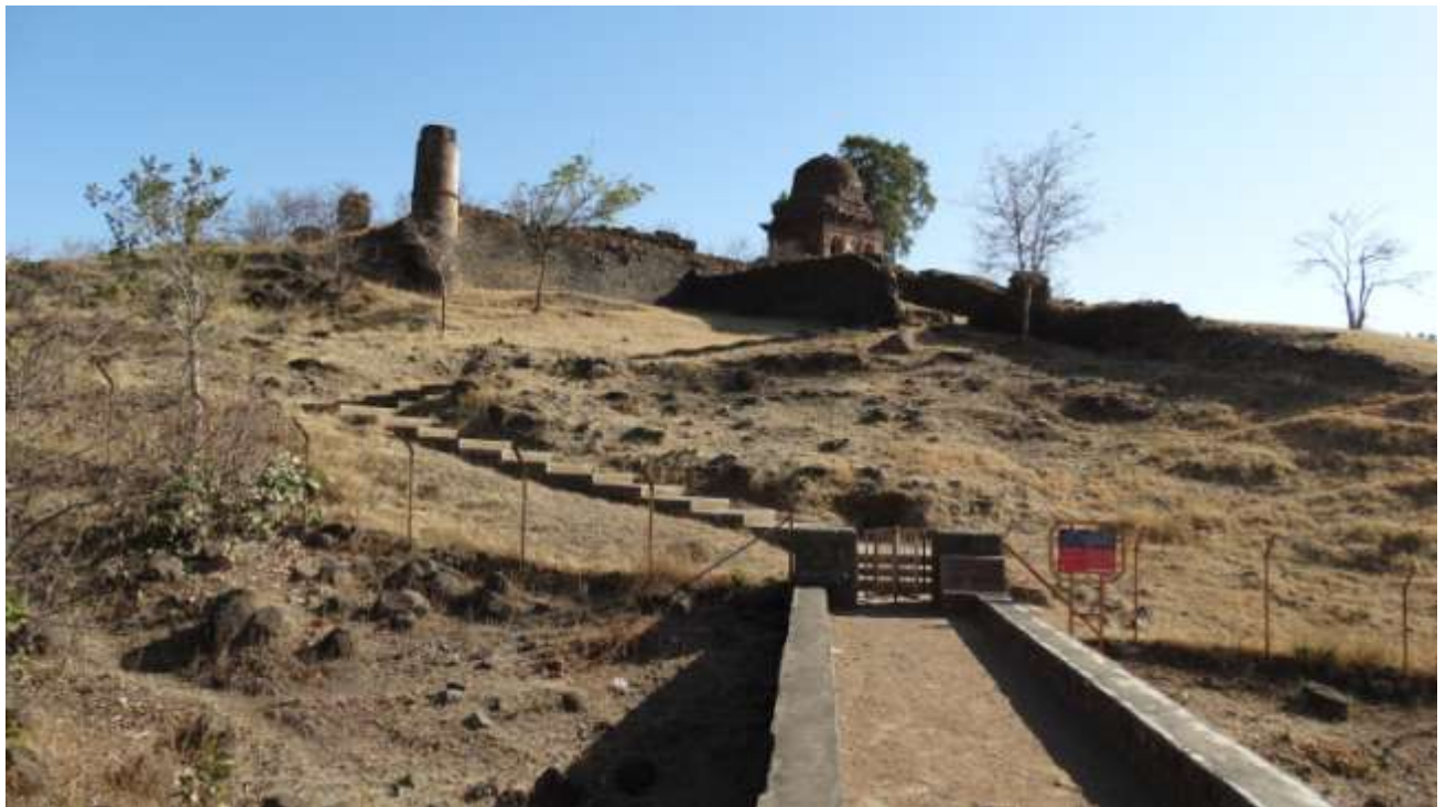
Plate 181 – Jali Mahal (before Alamgir Darwaza)
