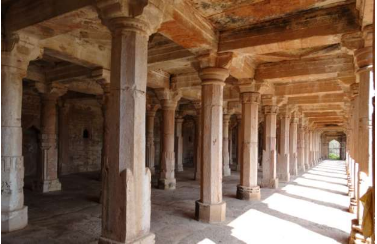
Plate 30 – Western wall of Dilawar Khan's mosque
