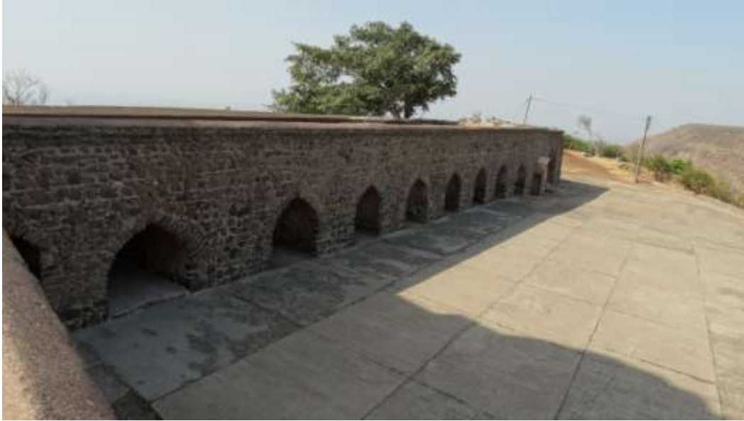
Plate 72 – the western extension of Rupmati pavilion
