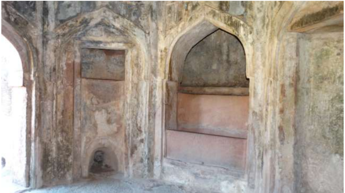
Plate 33 – western wall of the closed hammam from inside
