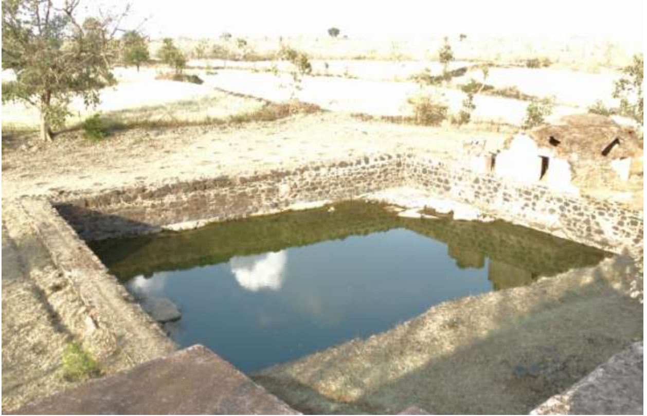
Plate 178- water tank in compound of Lal Bangla
