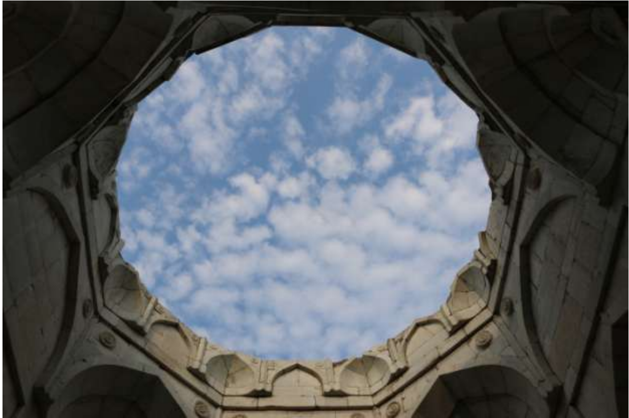
Plate 129 – the roof of the porch
