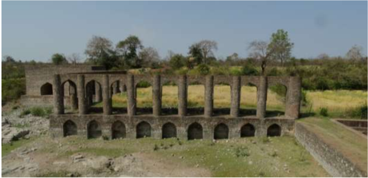
Plate 43 – Aqueduct behind Jal Mahal
