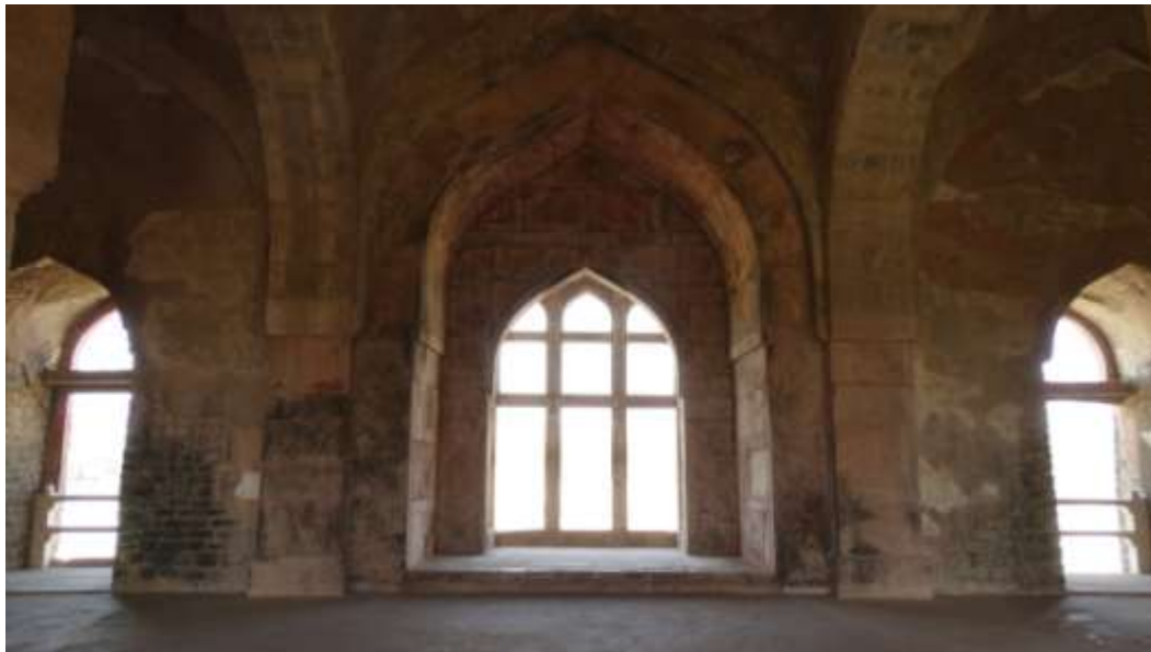
Plate 5 – western wall of the double hall of Jahaz Mahal
