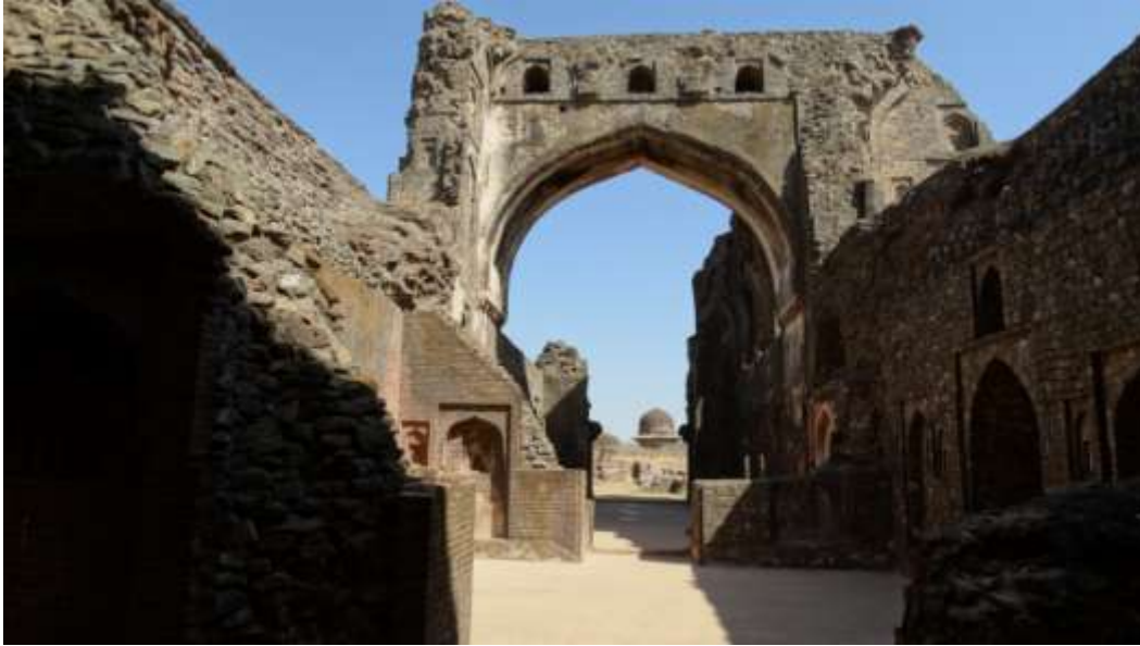
Plate 50 – Public Structure (Gada Shah’s shop)
