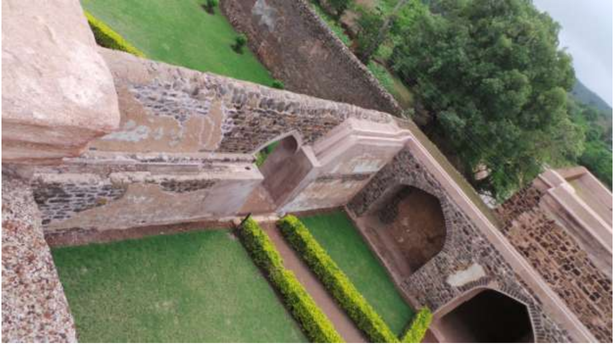
Plate 79 – water carrying channels along the southern wall of the courtyard of Baz Bahadur palace.
