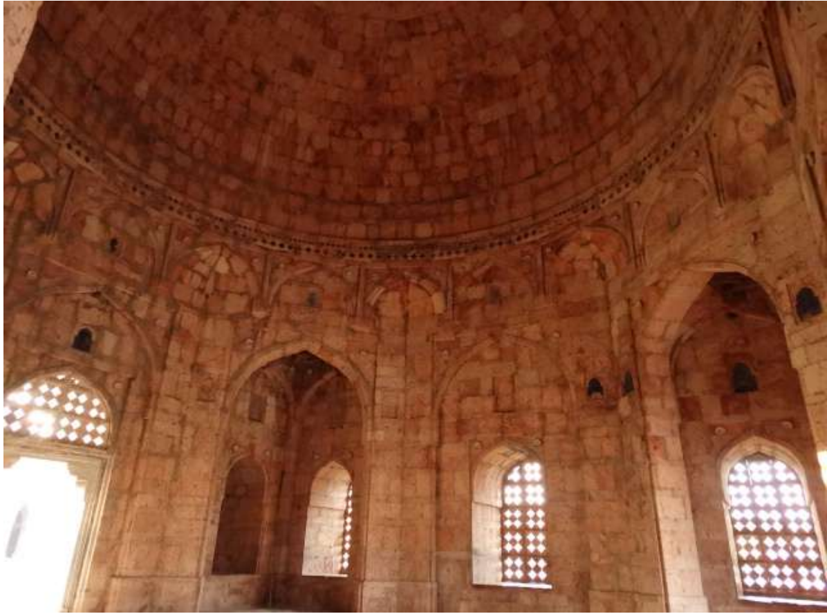
Plate 110 – interiors of the Jami Masjid Porch
