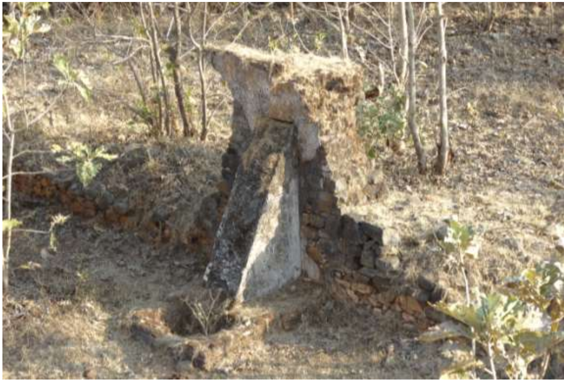
Plate 179- water carrying channels in Lal Bangla compound
