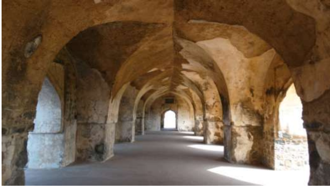
Plate 70 – the hall of the first floor
