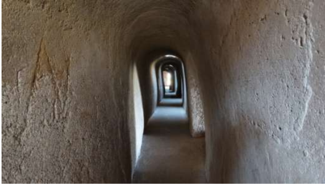
Plate 81 – passage behind the tank of the western extension of Rupmati Pavilion
