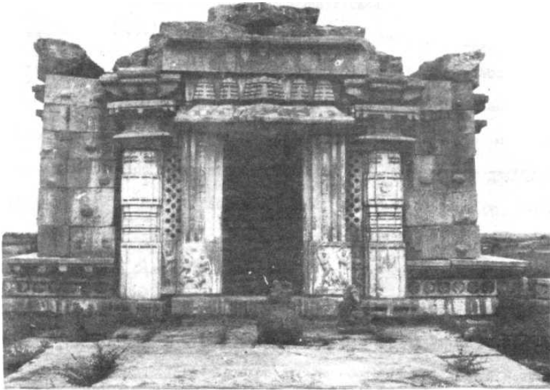
Period IV: Provision of stone bulbs on the walls used to lift and lead the stone during Temple construction, Kusumanchi, Sub-region B
