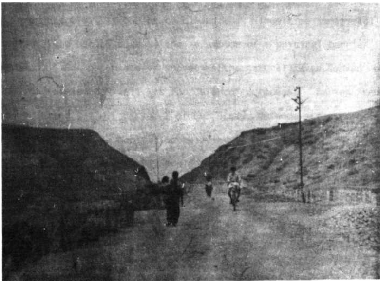
Period IV: Earthen rampart, Warangal, Sub-region B
