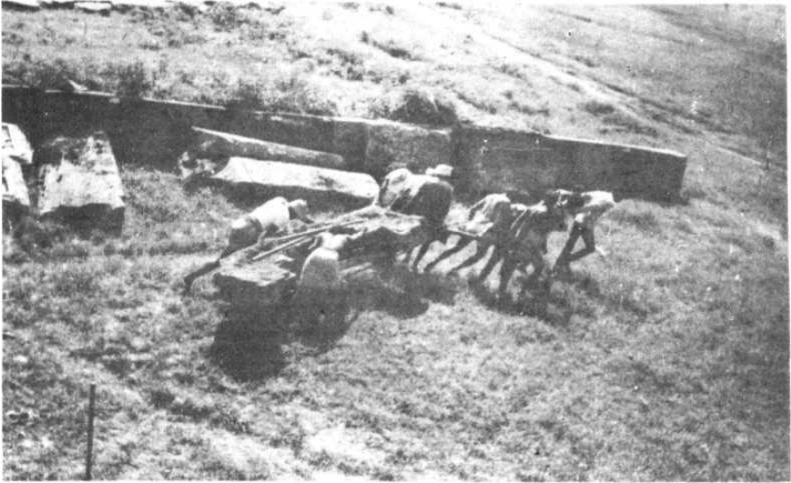
A small wooden cart drawn by men to transport the Temple Vargams within the site, Ramanujapur, Sub-region B
