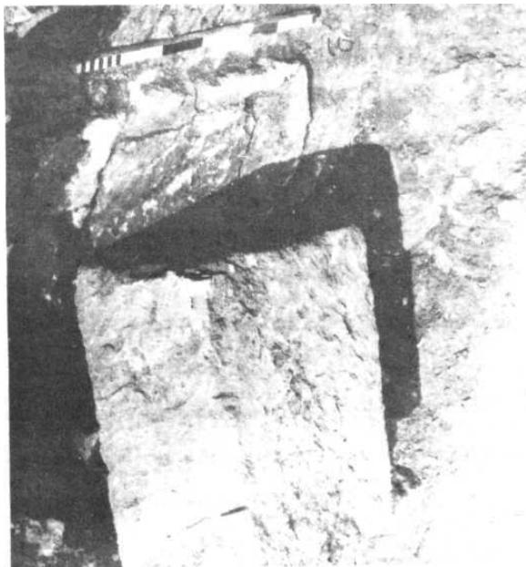
Period II: Foundation of a pillar in 'under pinning technique', Thotlakonda
