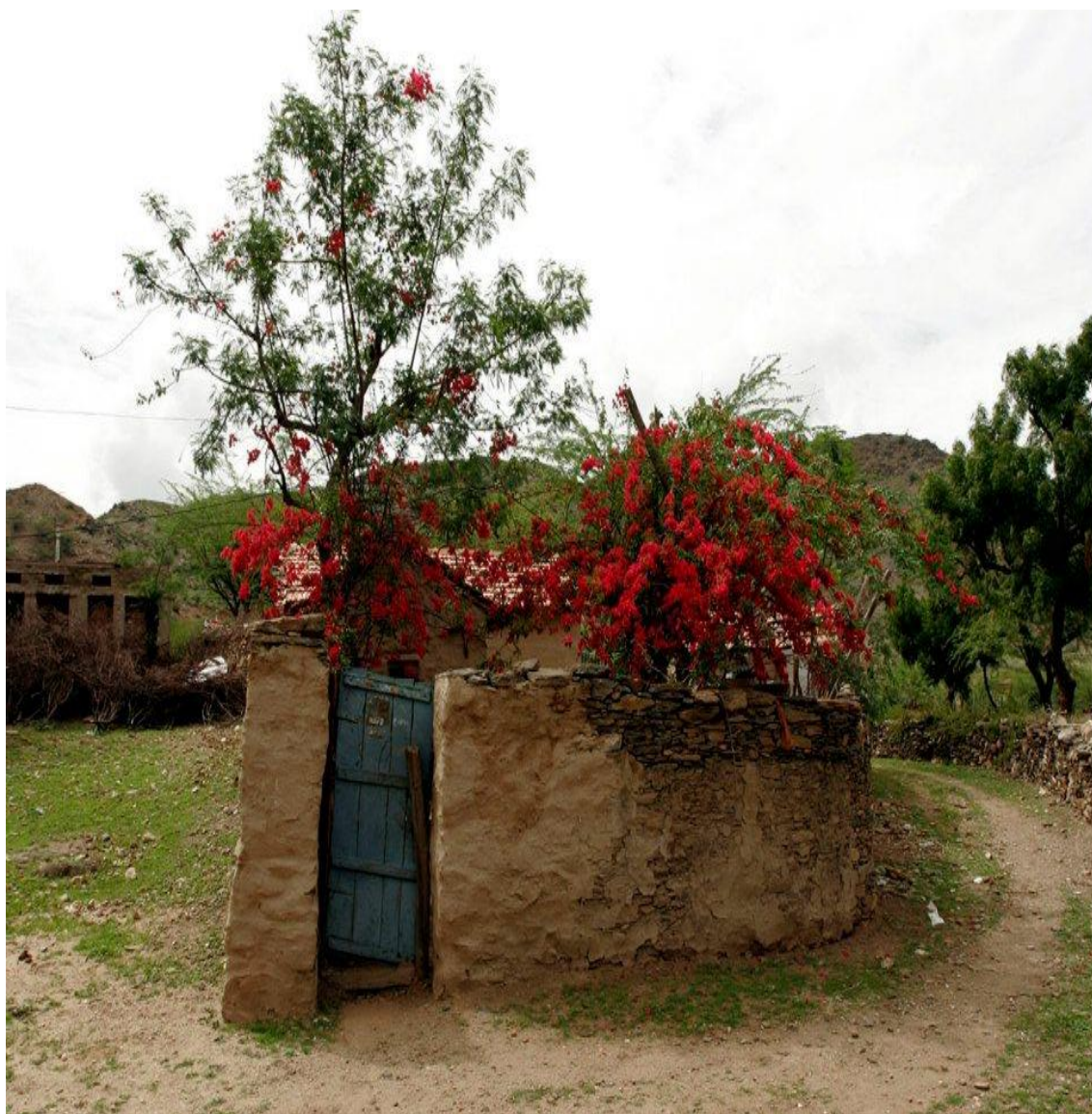
Figure 5.1: Mud House—MKSS Home and Office at Devdungri
