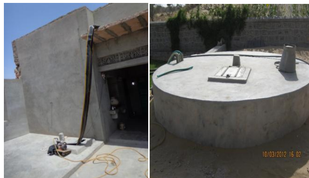
Photo 4.6. Tanka , Rain water harvesting from the house roof. Photo captured by the researcher during the field work
