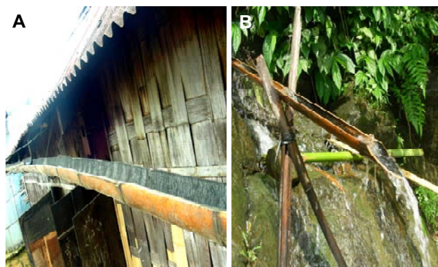
Fig. 9 Bamboo pipes. (A) Pipe for rain water collection from the roof top. (B) Collection of water from running river.
