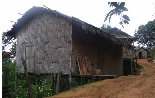
Fig. 2 Mizo typical bamboo house made from Melocanna baccifera and other bamboo species.
