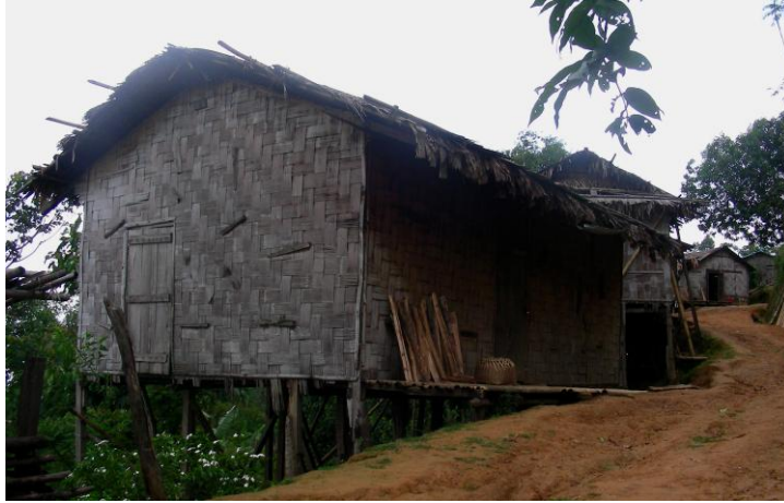
Figure 65. Mizo typical bamboo house made from Melocana baccifera and other bamboo species
