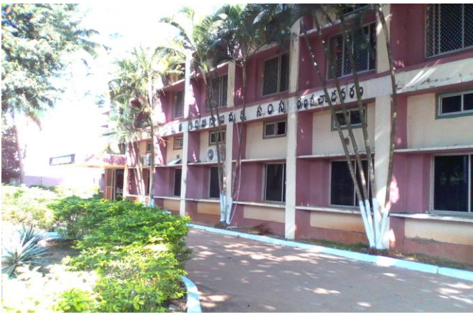
ITDA Office, Rampachodavaram
